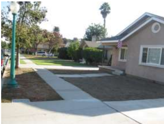
Before: Inadequate landscape in front yard areas.
