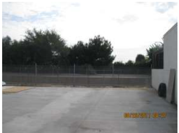
After: Removed trash, junk and debris.
