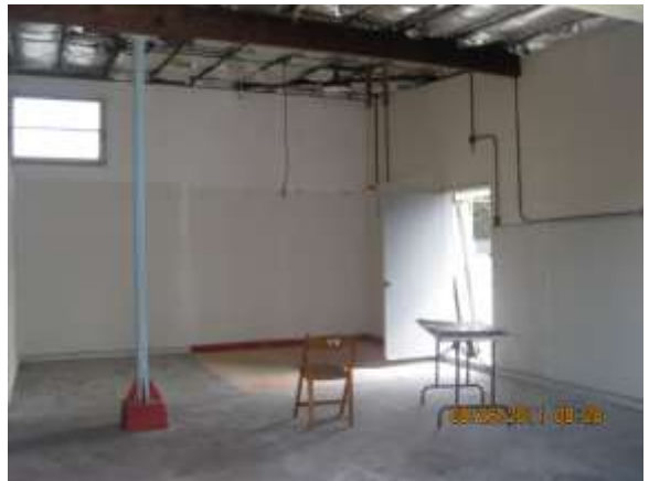
After: Living quarters removed.
