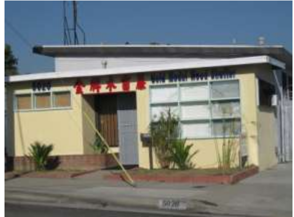
After: Front wall/façade painted and signage installed.
