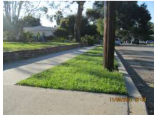
After: Adequate parkway after sod installation.
