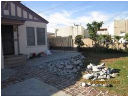
Before: Concrete extension being removed.
