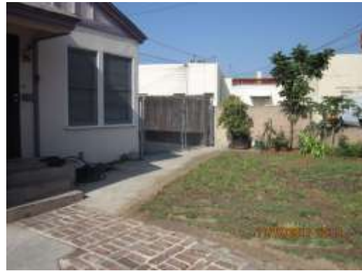
After: Concrete extension removed.
