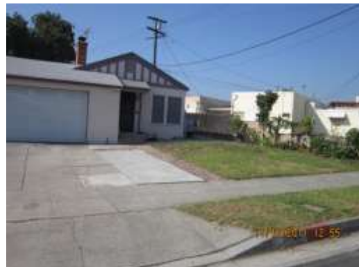
After: Concrete extension removed.
